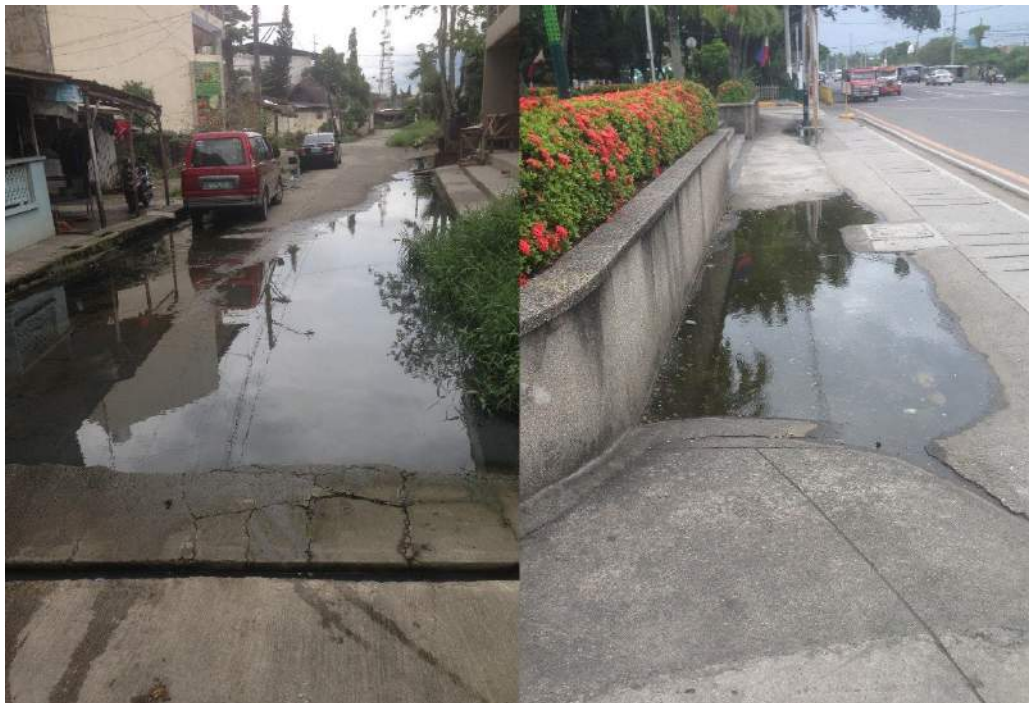
Figure 15. Pooling water and flooded streets in Malolos. Source: Leanna Leib-Milburn.
